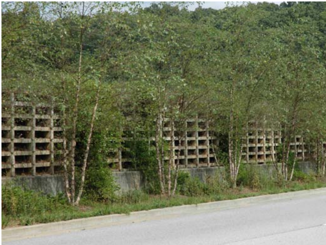
Interlocking block wall with landscaping Cumberland Blvd – Cobb Co., GA
