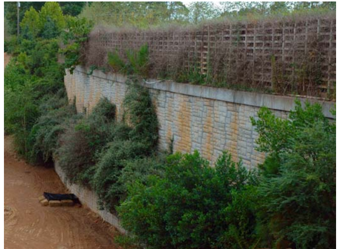
Terraced retaining wall with landscaping Cumberland Blvd – Cobb Co., GA
