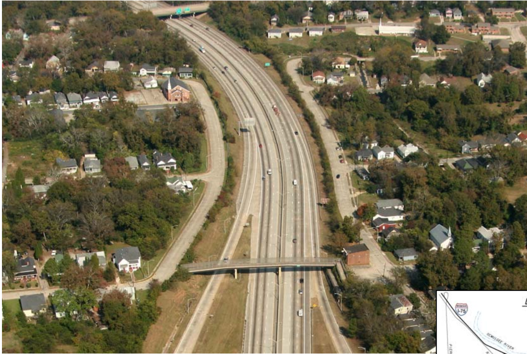
I-75 looking northbound - Before
