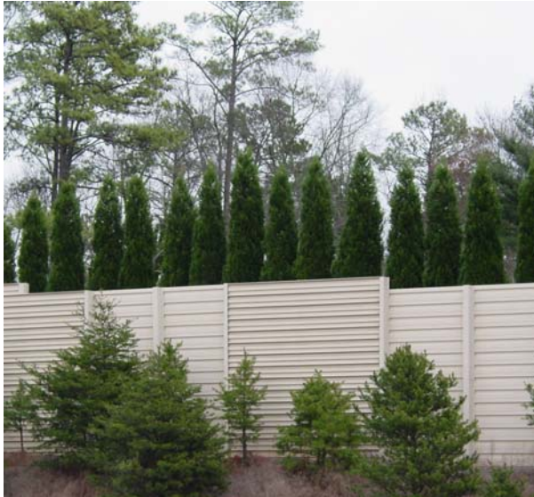
Standard steel barrier with landscaping added to improve aesthetics.
